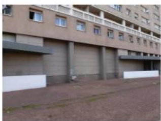
EXISTANT (FACADE EST)
